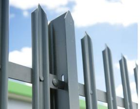
Fence detail:Pale,post,rail bolt and fish plate
